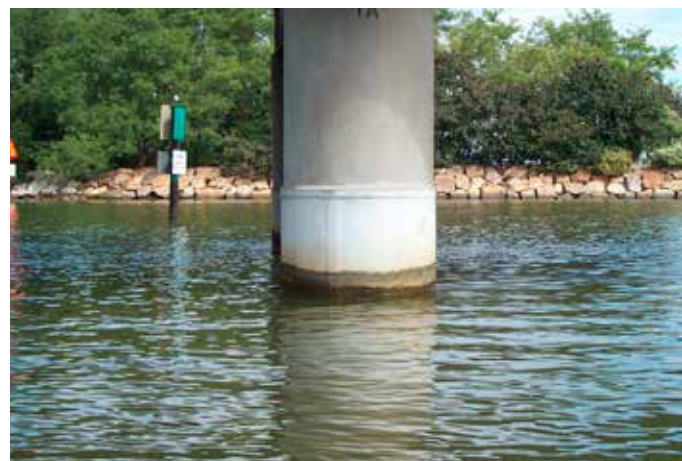
Close up of FX-70® repair to Bent #1A; in service 30 years
