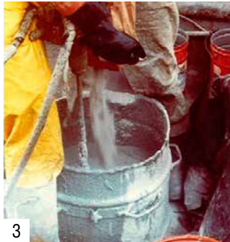
▲ FX-70®-6MP grout mixed in work boat
