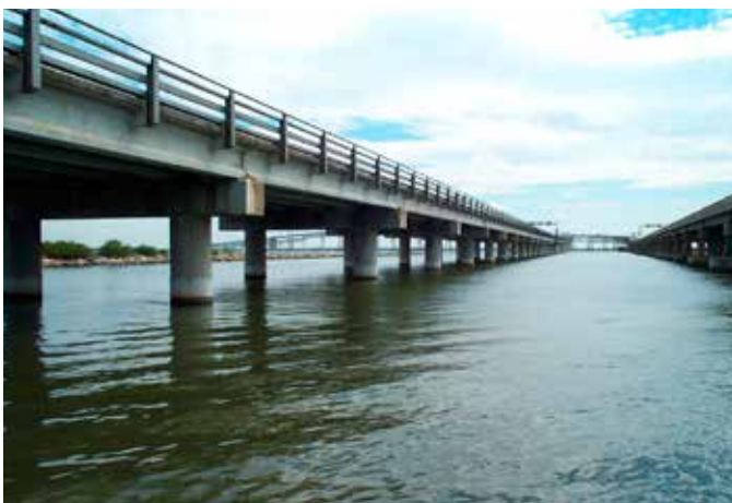
View of piles repaired with FX-70® System on western shore approach
