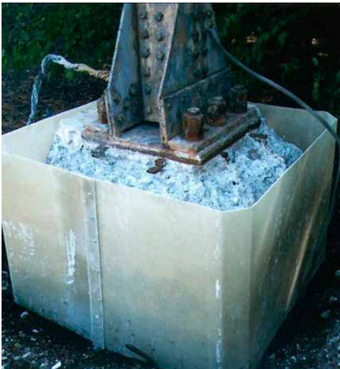
FX-70 jacket installed and backfilled
