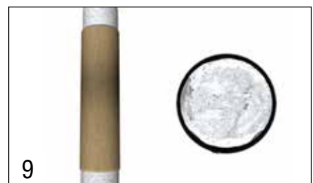
9 Remove ratchet straps. Repair complete.
