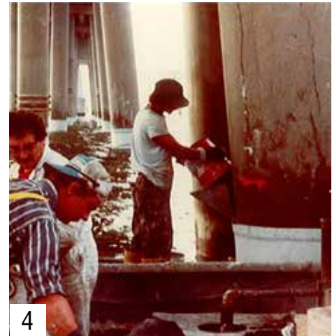
▲ FX-70®-6MP grout placed in jacket without dewatering
